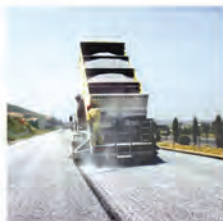
16 / 橡胶沥青同步碎石封层技术 SYNCHRONOUS CHIP SEAL WITH ASPHALT RUBBER
