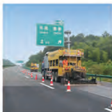
32 / MOH材料处理桥头跳车技术 MOH MATERIALS FOR TREATING THE BUMPING AT JOINTS OF BRIDGE-ROAD
