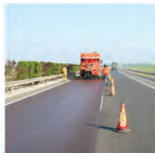
06 / 低噪声微表处技术 LOW-NOISE MICRO SURFACING
