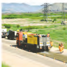
18 / 纤维碎石封层技术 FIBER-REINFORCED CHIP SEAL
