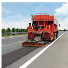
08 / 微表处修复车辙技术 RUTS REPAIR BY MICRO SURFACING
