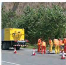
30 / MOH材料路面坑槽修补技术 MOH MATERIALS FOR PIT SLOT REPAIR
