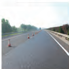
12 / 纤维微表处技术 FIBER- REINFORCED MICRO SURFACING
